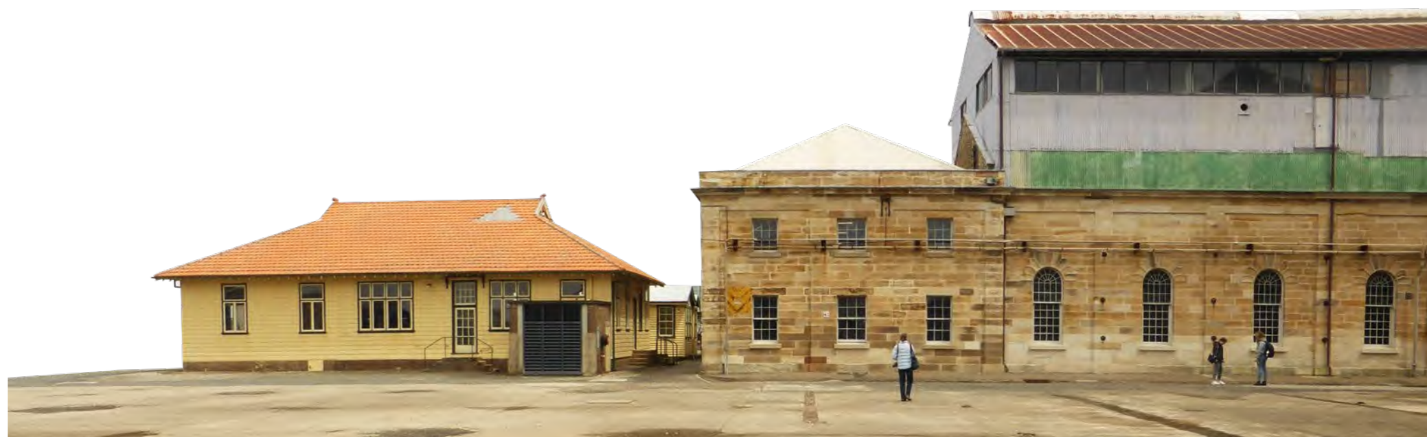
Fig 42. One of the most important elevations of the Convict Workshops, with subsequent layers of maritime use in starkly different materiality and form. Source: Tyrrell Studio
