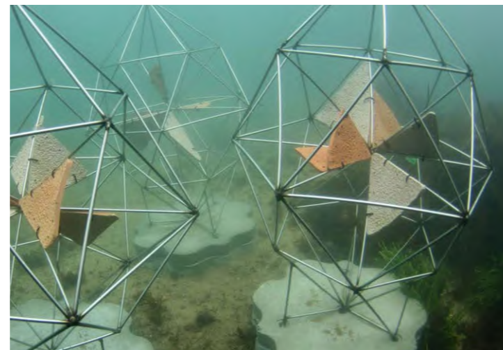
Fig 77. Artificial reefs can be formed from various materials including marine-grade steel or concrete. Source: Reef Design Lab and SIMS
