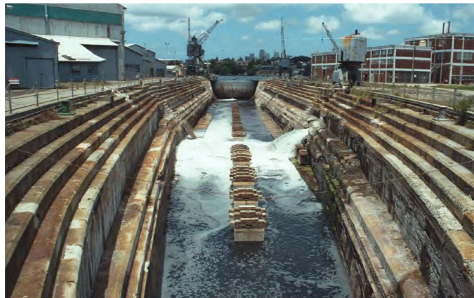
Fig 99. Fitzroy Dock being refilled is a dramatic show of the engineering marvel of the docks. Source: John Jeremy
