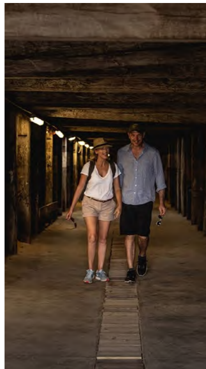
Fig 69. The Dog Leg Tunnel. Source: Sydney Harbour Federation Trust
