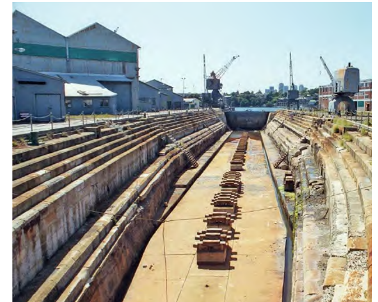
Fig 96. Drained Fitzroy Dock. Source: John Jeremy
