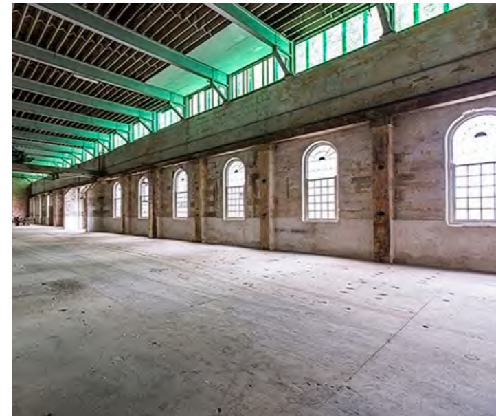
Fig 91. The interior of the Convict Workshop. Source: Sydney Harbour Federation Trust
