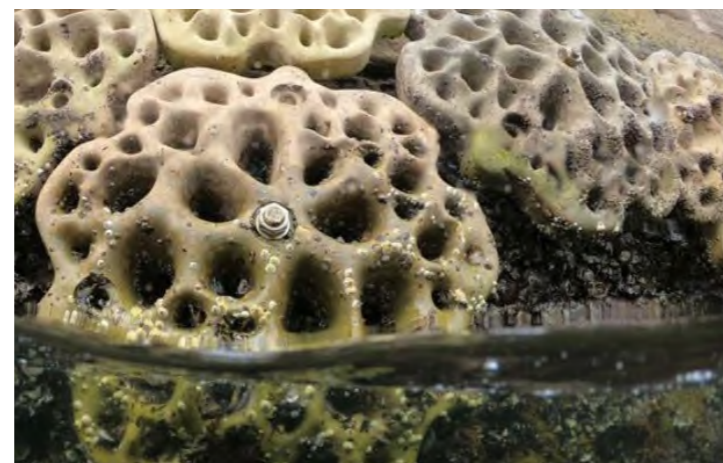
Fig 78. Precast concrete tiles provide natural habitat against typically flat seawalls. Source: Reef Design Lab and SIMS
