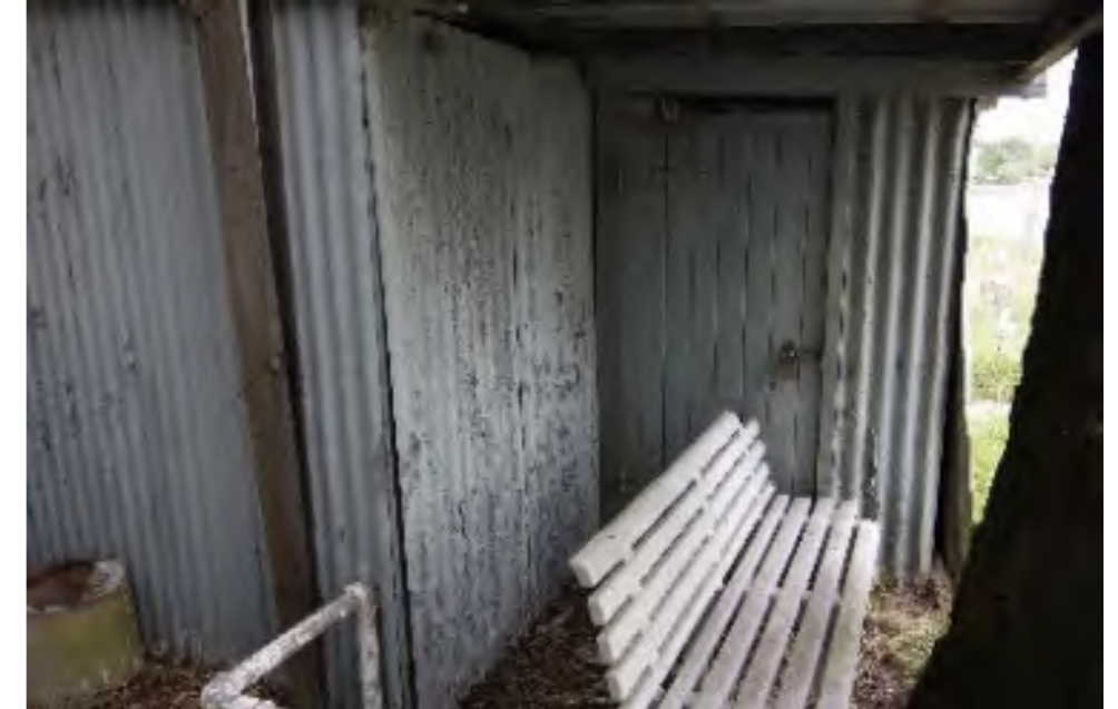
Fig 26. Site conditions. Source: ERM
