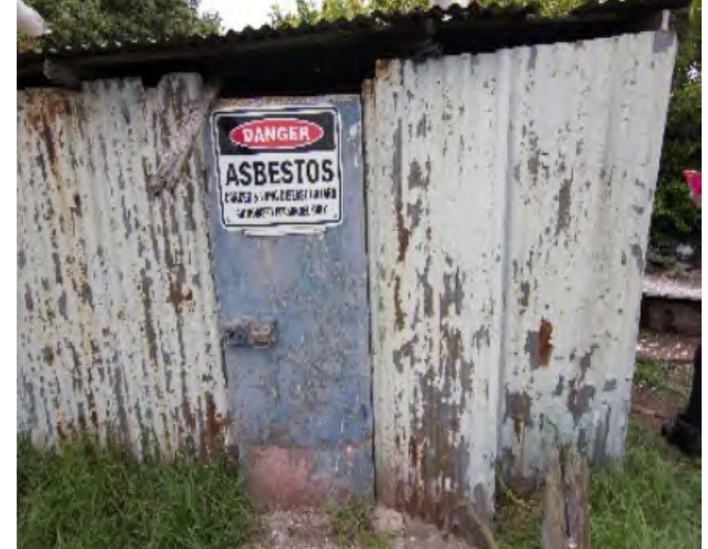
Fig 28. Site conditions. Source: ERM
