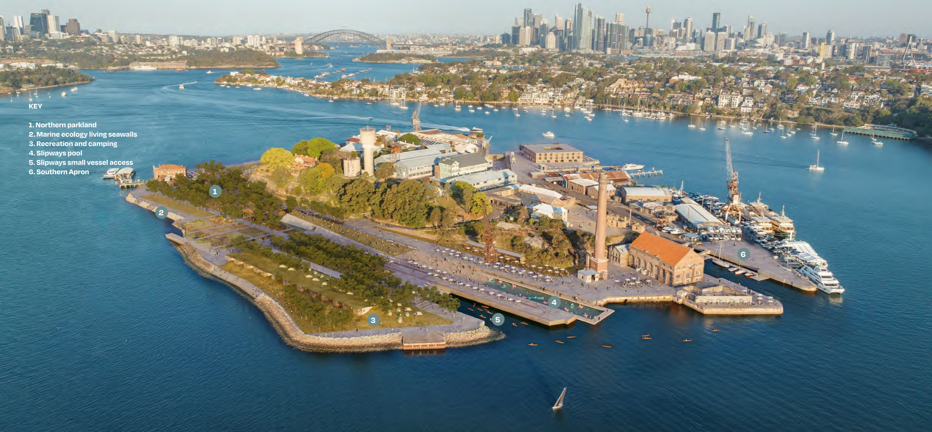
Fig 7. Artist impression of the master plan aerial view looking east . Source Tyrrell Studio/Doug & Wolf
